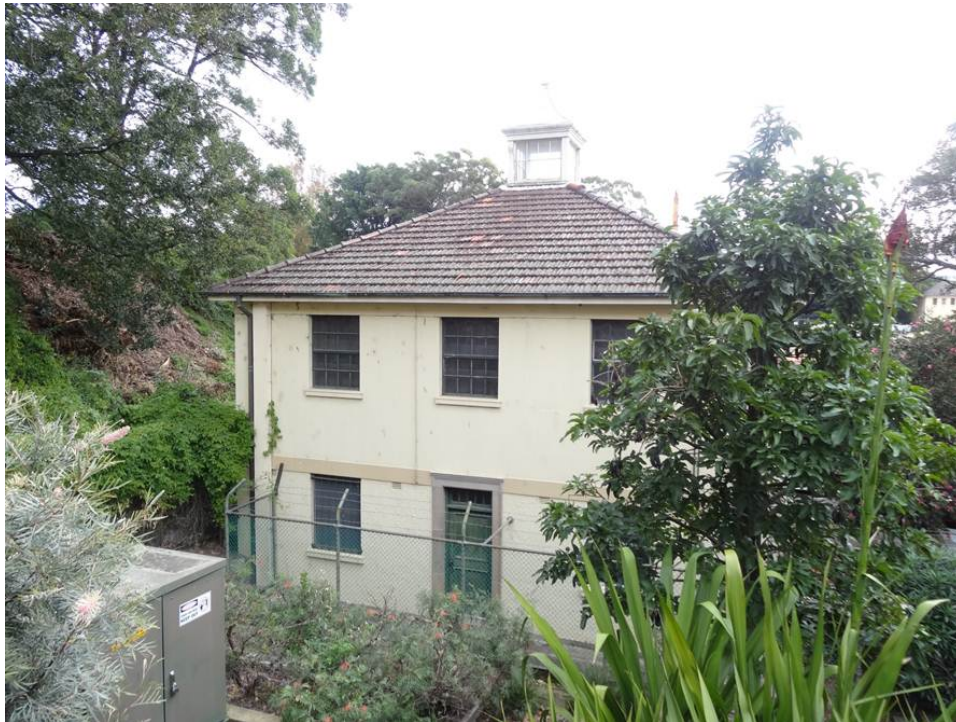
Figure 26: Existing Animal House to be demolished
