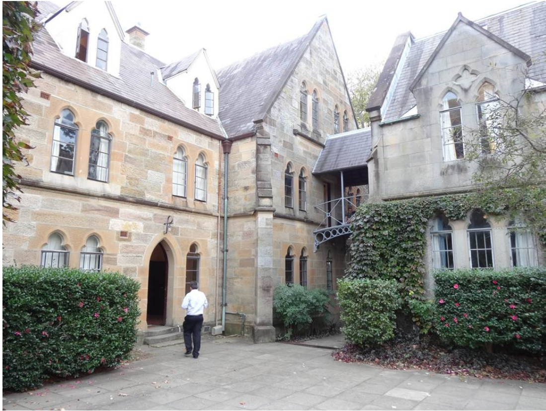
Figure 7: Existing Garnsey Wing viewed from Old Quadrangle
