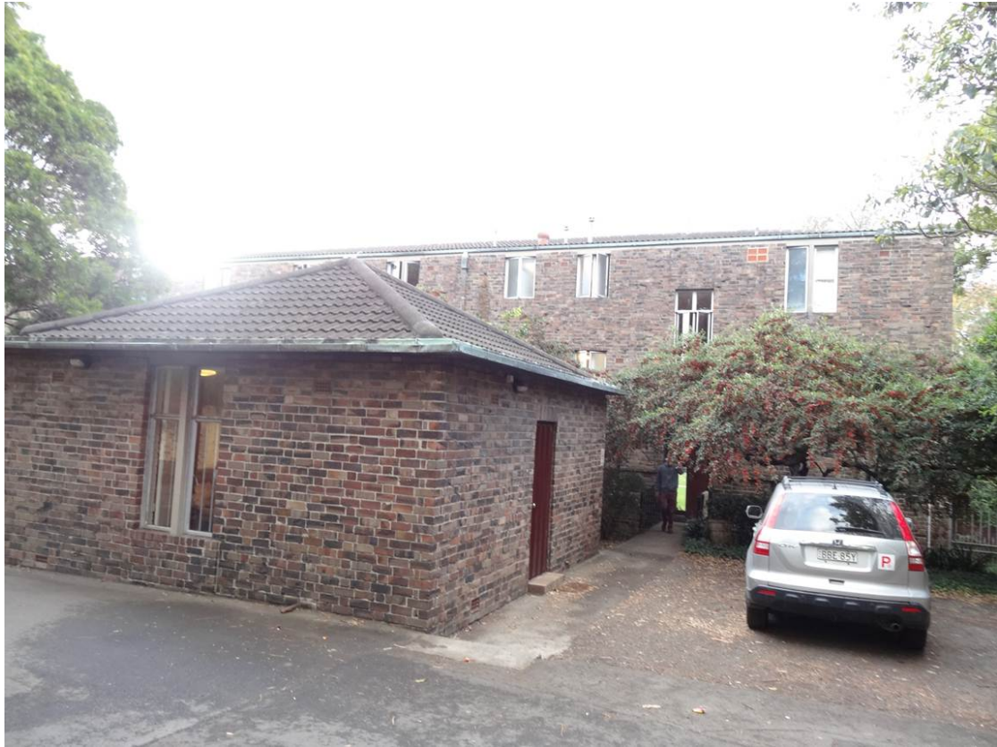
Figure 9: Existing Arnott Building and single storey annexe
